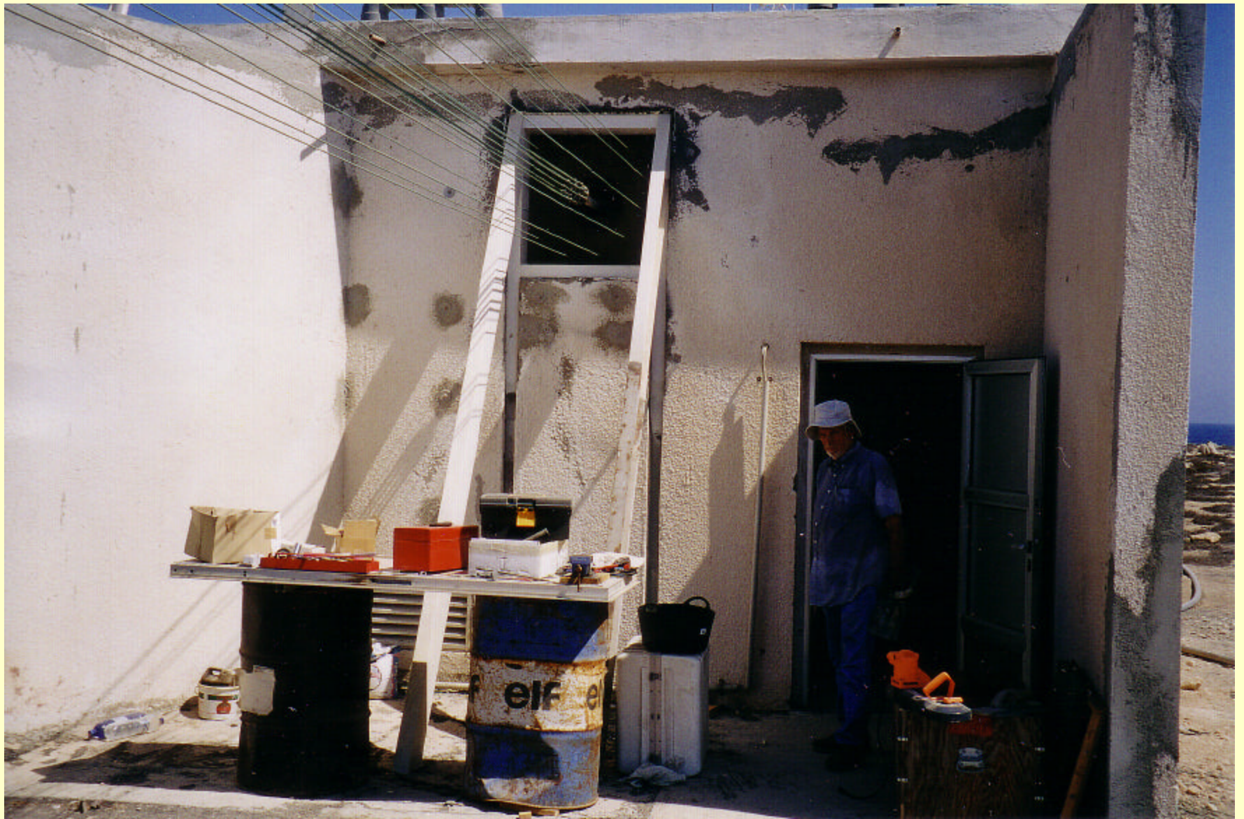
WORK UNDERWAY AT ANTENNA EQUIPMENT BUILDING
