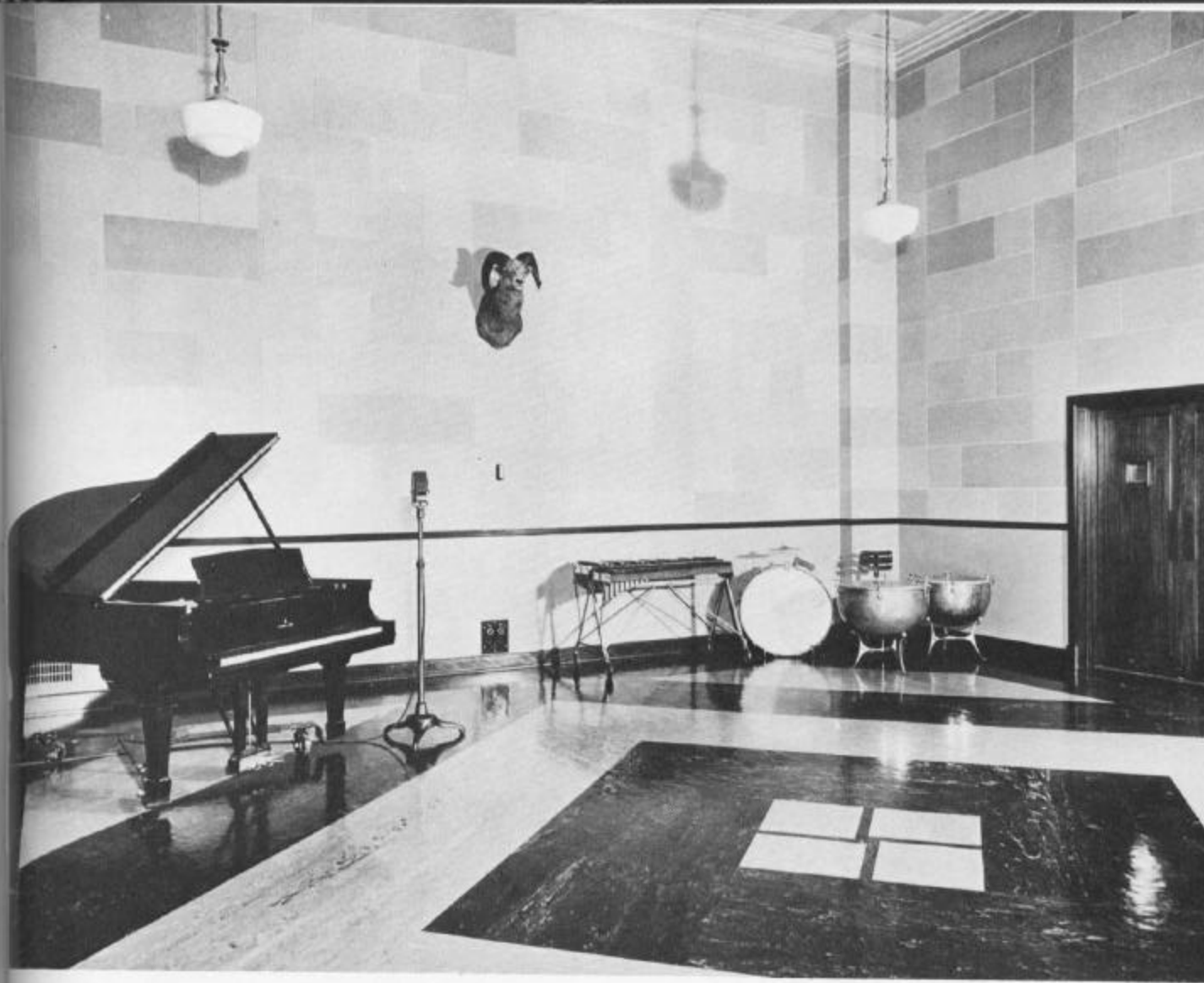
(Seattle Historical Society) Studio "B," one of four deluxe studios built for KOMO-KJR 's combined operation on the seventh floor of the Skinner Building in Seattle, July, 1933. The construction was something marvelous. Floors floated on six inches of balsam wool. Walls, doors and ceilings were double; and glue, rather than nails, held things together. It was one of the finest broadcast installations in the world.
